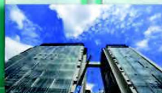
West Kowloon Law Courts Building
